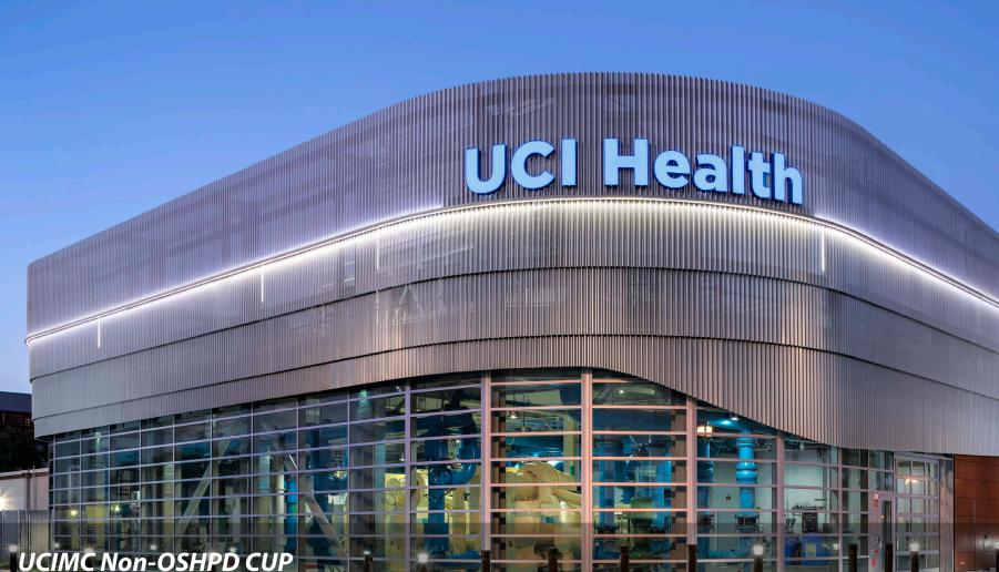
The Non-OSHPD CUP and electrical pl g at the entrance to campus. The team exceeded client expectations with a beautiful open storefront concept utilizing buckling restrained braces and a steel gravity system.
